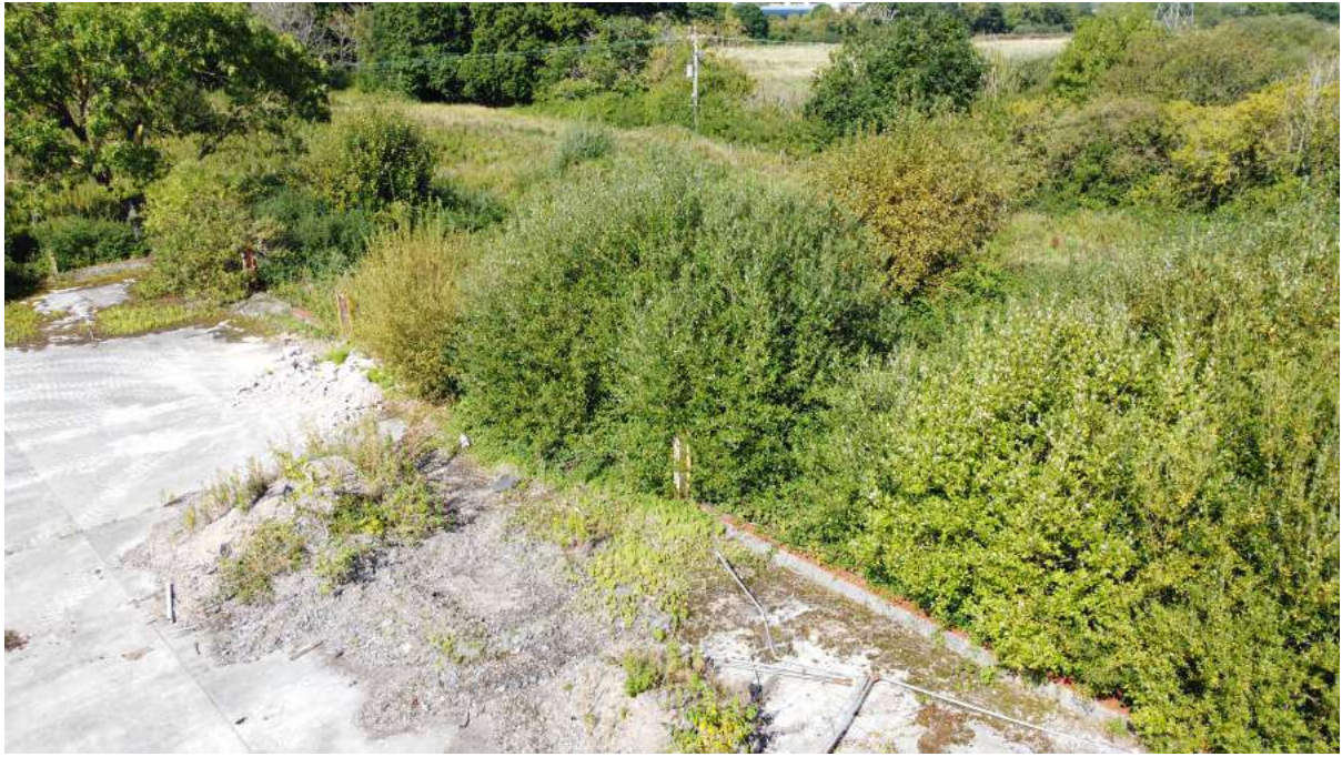
Partially obscured retaining wall & Steel Stanchions.
