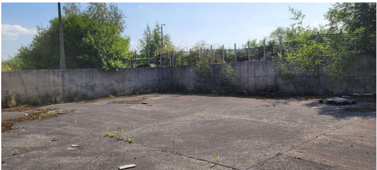
Reinforced Concrete Wall
