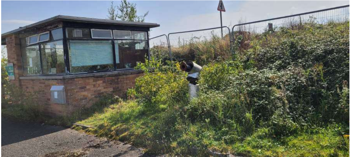
Former Gate House – Note Steam Pipe
